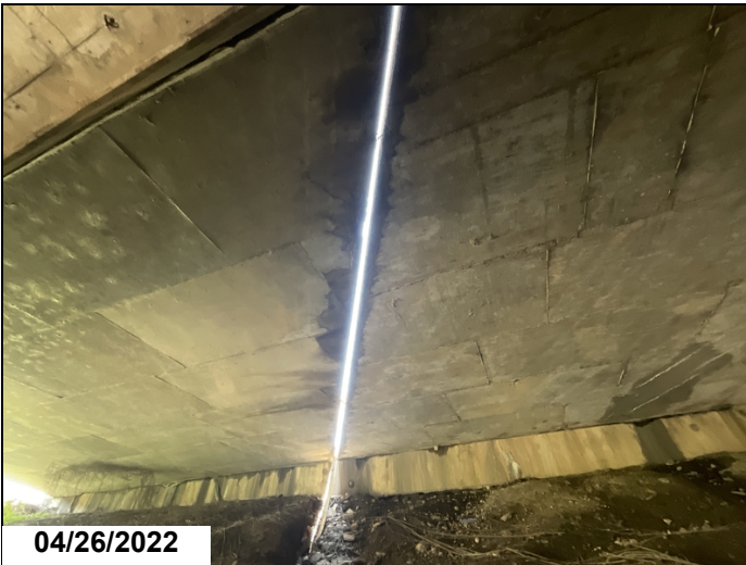
Slabs have up to four inch+ gap between left and right slabs in span #1 and up to two inches in span #2.
