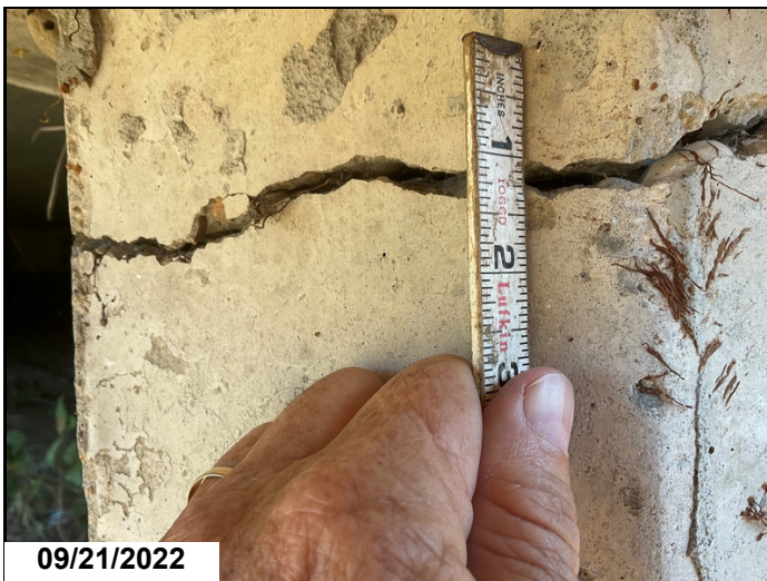
1/4" crack in bent #2 pile #12
