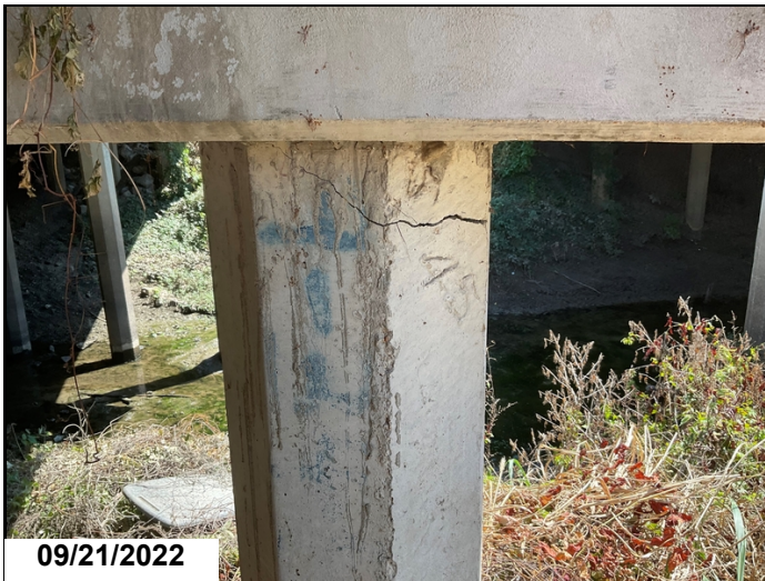
1/4" crack in bent #2 pile #12
