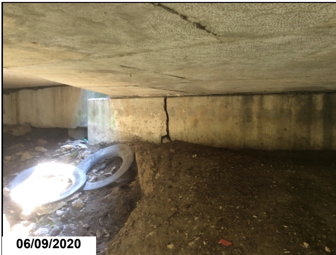
Abutment 2 left end crack.
