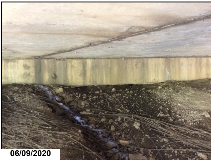
Abutment 1 cap undermined.
