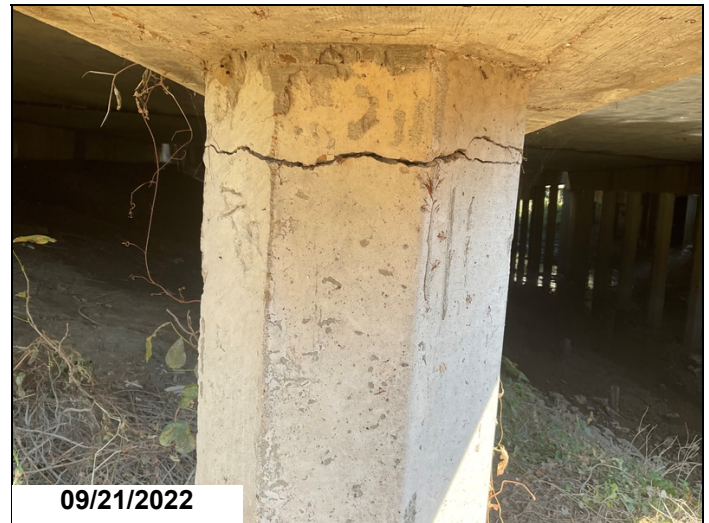
1/4" crack in bent #2 pile #12
