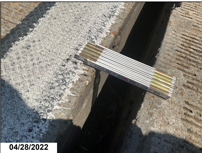
Width of gap between right and left slabs near abutment #1.
