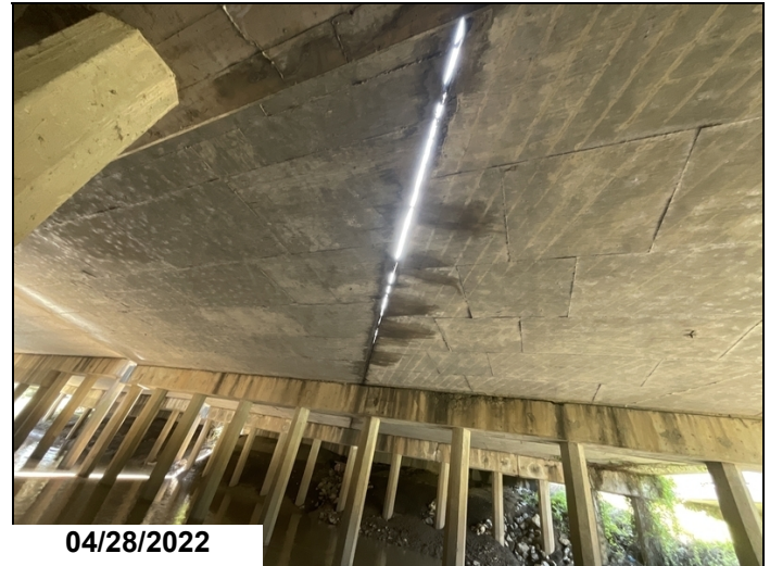
Span #2 under side of deck at joint between right and left slabs.
