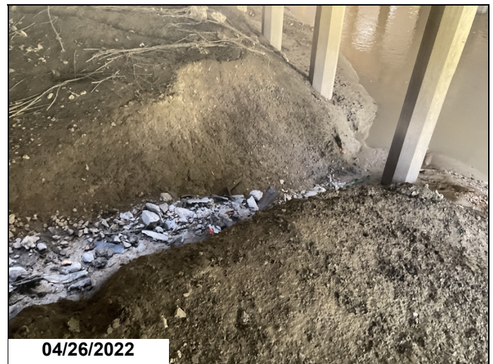
Abutment #1 slope erosion between piles #6 and 7.
