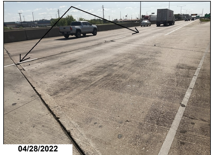
Length of gap between spans
