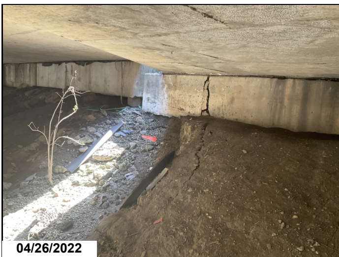
Abutment #2 cap left side cracked and slope eroded.
