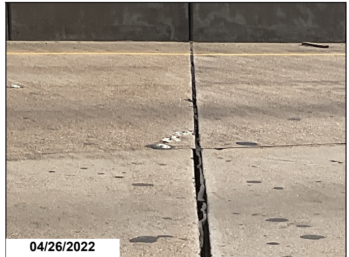
Bent #3 span #2 at center line has two foot cracked / delaminated area.
