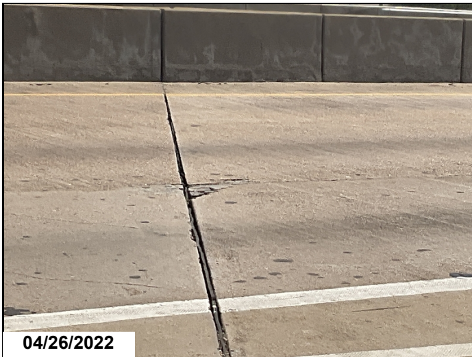
Span #4 bent #4 at center line has two foot patched area
