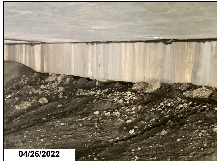
Abutment #2 cap undermined for fifteen feet at center line up to one foot exposing two piles.
