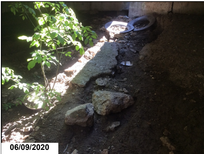
Abutment 2 left side has erosion up to 2' deep.
