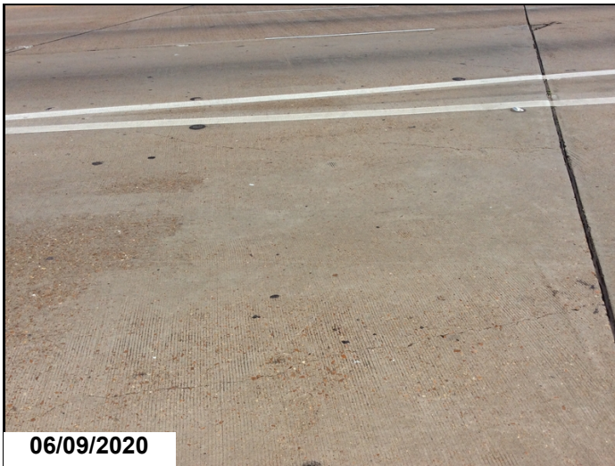
Typical deck crack.
