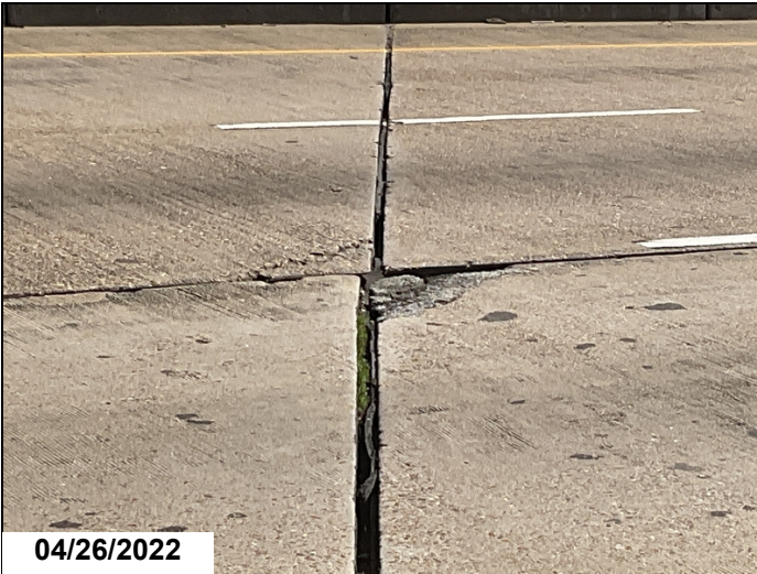
Bent #2 span #2 at center line has two foot cracked / delaminated area, span #3 has patched area
