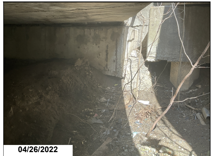
Abutment #1 cap left end undermined up to six inches for one foot.
