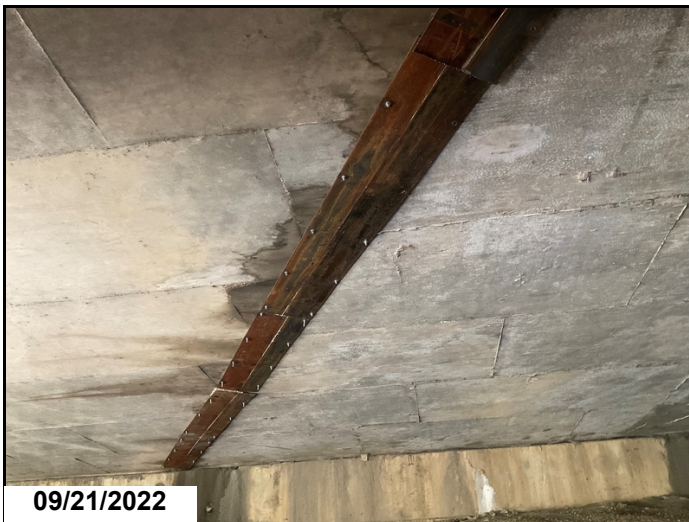
Span #1 soffit / underside of deck at slab separation repair
