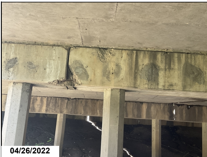
Bent #3 cap between piles 9,10 has a spall with exposed rebar on ahead face and one foot shallow spall with no exposed rebar.
