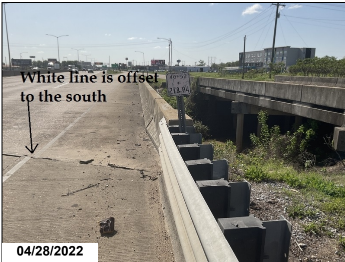
Abutment #1 right white line offset due to right half of slab rotating to the south.
