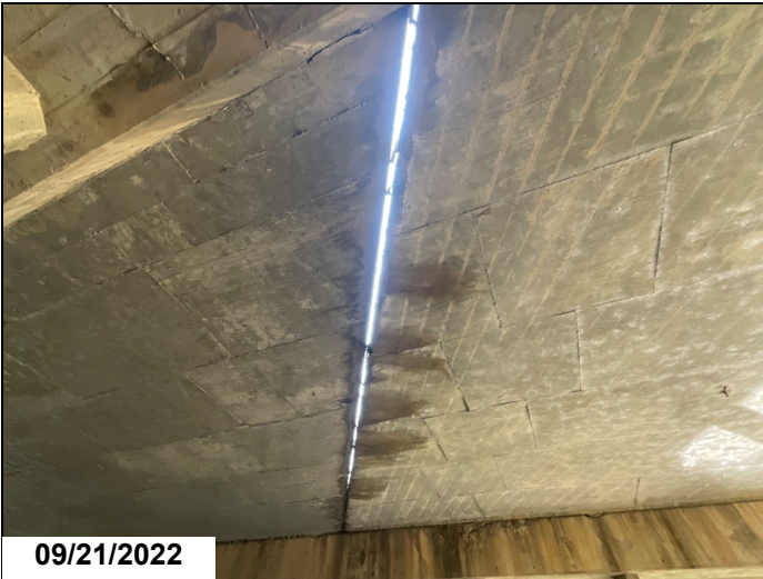
Span #2 soffit between slabs approximately 2" gap at bent #2
